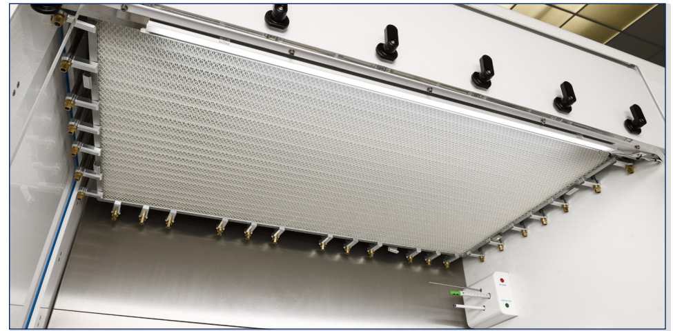
HEPA Filter located in the ceiling
